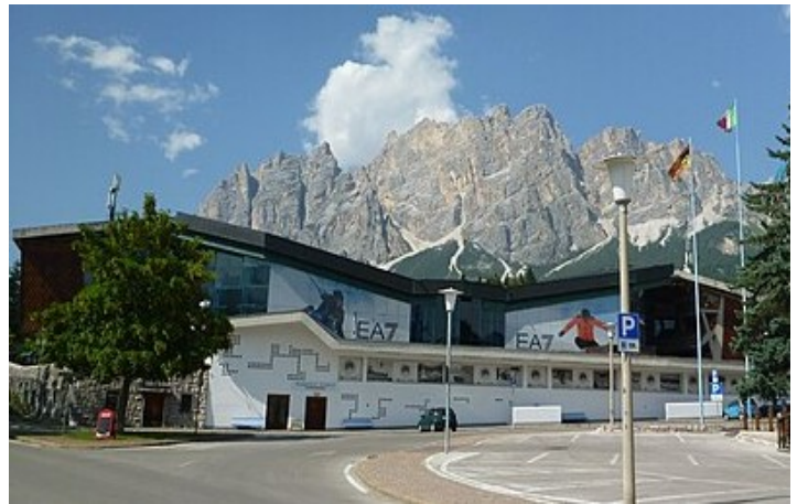
Cortina Curling Olympic Stadium
